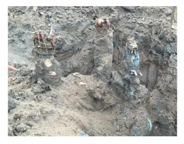
Figure 9 – Verification of the integrity of micropiles. Source: Author (2016)
