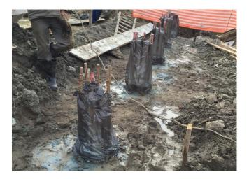
Figure 10 - Top of piles after demolition of excess cement. Source: Author (2016)
