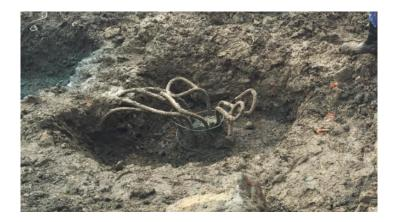
Figure 11 – Heavy machinery circulated over the micropiles. Source: Author (2016)
