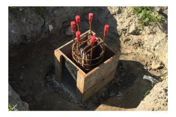
Figure 5 – Connection between piles and pile caps. Source: Author (2016)
