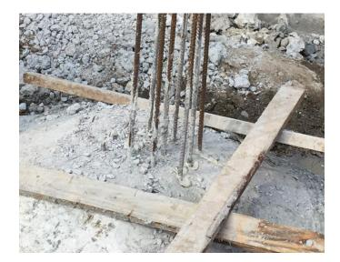
Figure 3 – Inappropriate solution for footing location correction. Source: Author (2016)
