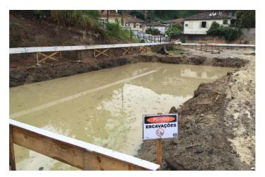
Figure 2 – Flooding on Block 4 excavation. Source: Author (2016)
