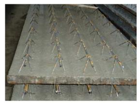
Figure 3 - metal template with concrete and lattice.
